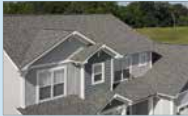
Roofing and Ventilation
